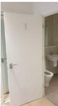
Captured (certified by inspector): 01/04/19 Added: 04/04/19
