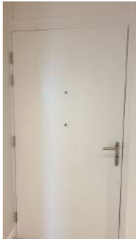
Captured (certified by inspector): 01/04/19 Added: 04/04/19
