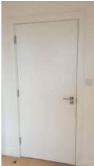
Captured (certified by inspector): 01/04/19 Added: 04/04/19
