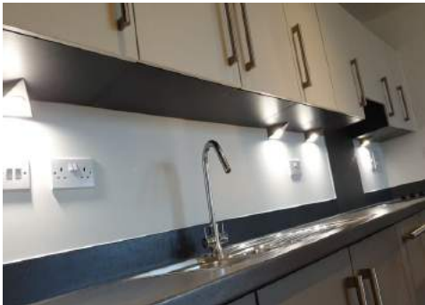
Captured (certified by inspector): 01/04/19 Added: 04/04/19
