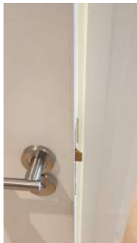
Captured (certified by inspector): 01/04/19 Added: 04/04/19
