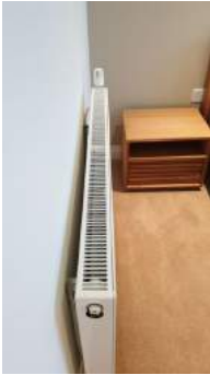
Captured (certified by inspector): 01/04/19 Added: 04/04/19
