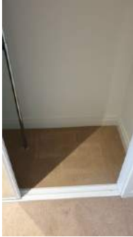
Captured (certified by inspector): 01/04/19 Added: 04/04/19
