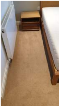
Captured (certified by inspector): 01/04/19 Added: 04/04/19
