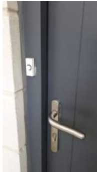
Captured (certified by inspector): 01/04/19 Added: 04/04/19
