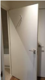
Captured (certified by inspector): 01/04/19 Added: 04/04/19
