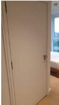
Captured (certified by inspector): 01/04/19 Added: 04/04/19
