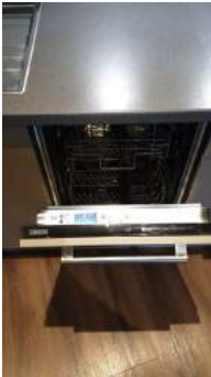
Captured (certified by inspector): 01/04/19 Added: 04/04/19
