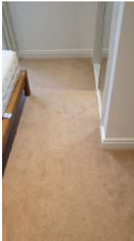
Captured (certified by inspector): 01/04/19 Added: 04/04/19
