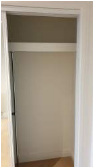
Captured (certified by inspector): 01/04/19 Added: 04/04/19
