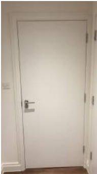
Captured (certified by inspector): 01/04/19 Added: 04/04/19
