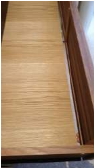
Captured (certified by inspector): 01/04/19 Added: 04/04/19
