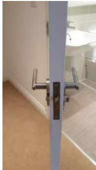
Captured (certified by inspector): 01/04/19 Added: 04/04/19
