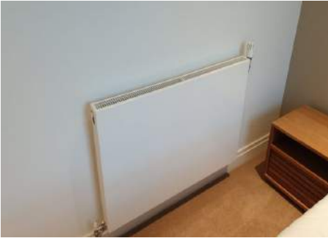
Captured (certified by inspector): 01/04/19 Added: 04/04/19
