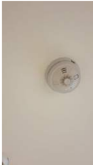
Captured (certified by inspector): 01/04/19 Added: 04/04/19
