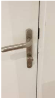
Captured (certified by inspector): 01/04/19 Added: 04/04/19
