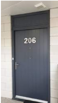
Captured (certified by inspector): 01/04/19 Added: 04/04/19
